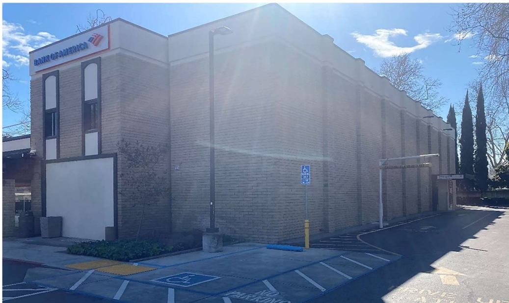
West façade, view facing southeast. Source: ESA, 2024.
