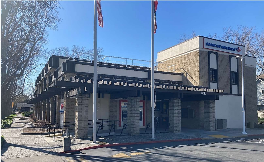
North façade, view facing south. Source: ESA, 2024.
