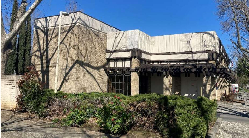
South façade, view facing northwest. Source: ESA, 2024.
